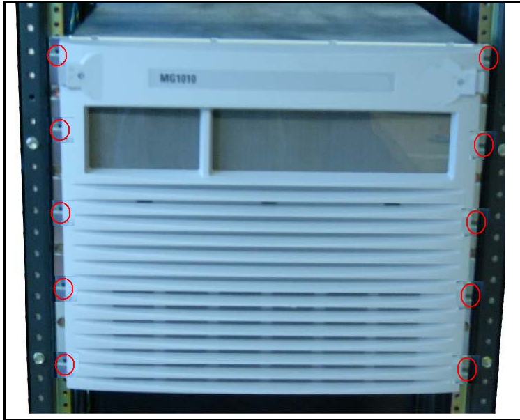
Figure 42 Media Gateway 1010 chassis screws
